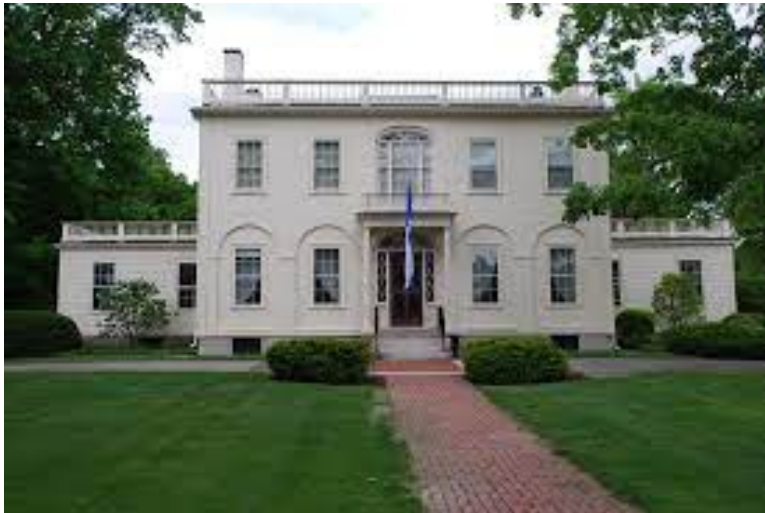
Known today as Phelps House, it was built in 1809-1812 with William Bartlet's money as housing for the Seminary's first Professor of Sacred Rhetoric, Edward Dorr Griffin. Andover Historic Preservation.
